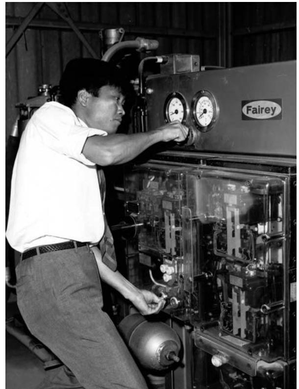
A student simulates miniature earthquakes transmitted to a "shaking table" by a hydraulic device, Tokyo, 1969. A United Nations Development Programme (UNDP) project for which UNESCO is the executing agency, collaborates with the Japanese government to train experts at the International Institute of Seismology and Earthquake Engineering to help developing countries combat the effects of earthquakes.
