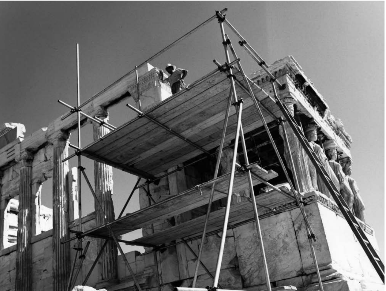
Restoration of the porch of the Caryatids at the Erechtheion, 1968. In 1977, UNESCO launched a campaign for the restoration and conservation of the Acropolis Monuments, which have been ravaged by centuries of war, earthquakes, fires, water damage, air pollution and mass tourism.
