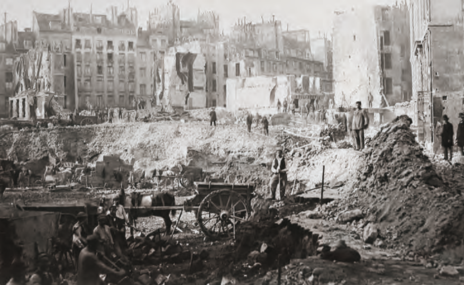
Major urban transformation works of Baron Haussmann on the Avenue de l'Opéra, Paris (France) © Charles Marville, 1862. Source: gallica.bnf.fr - Ecole nationale des ponts et chaussées*
